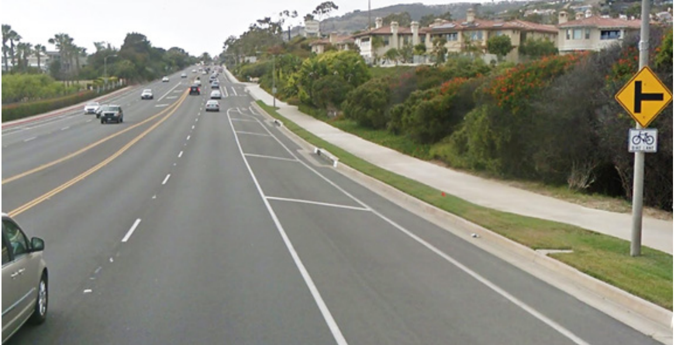
Travel Side Buffered Bike Lane on PCH (SR-1), Dana Point (Photo: Google Street View)
